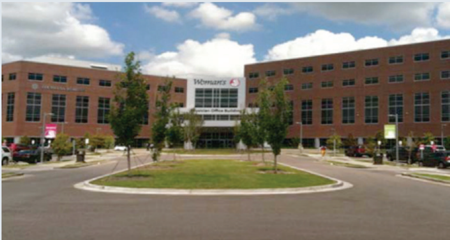
Woman’s Hospital Medical Office Building; Baton Rouge, Louisiana; photo by Rick Pearson
