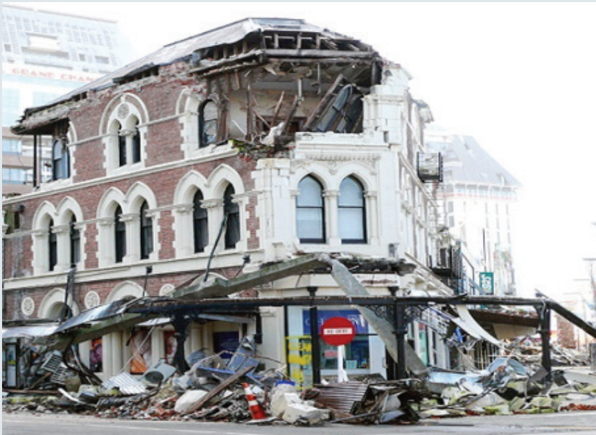
Earthquake damage assessment, Christchurch, New Zealand
